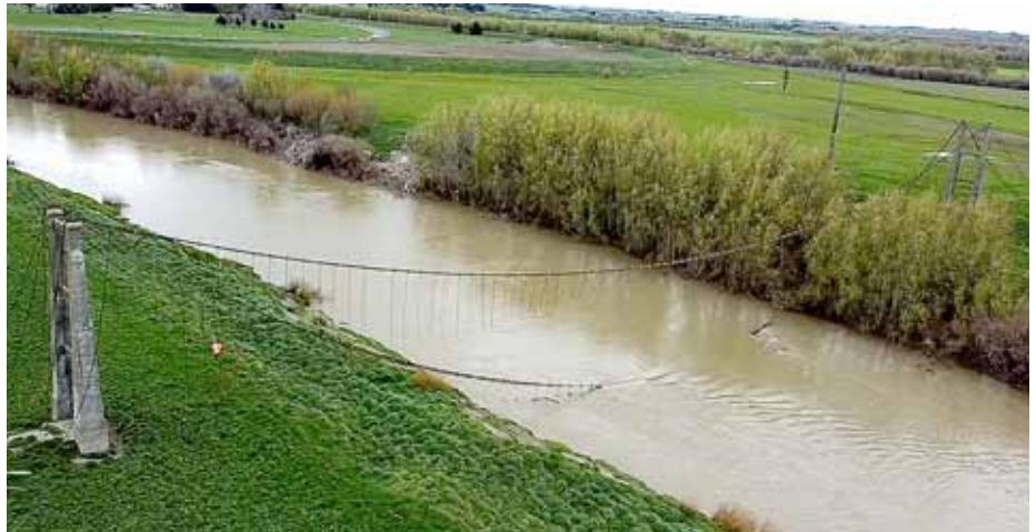
Opiki toll bridge after cable had fallen into the Manawatu river. Manawatu Standard/Stuff
