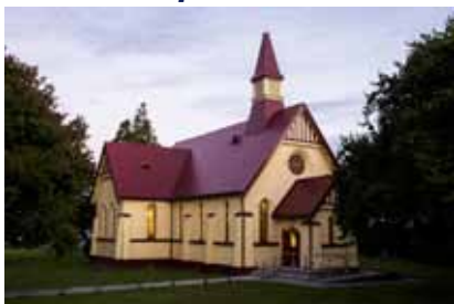
Toko Toru Tapu, Manutuke, Gisborne shows ordinary buttresses and angled buttresses. Strike Photography
