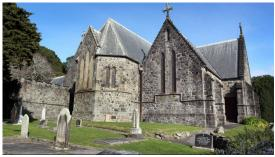
rods into the top then tie these tight with a concrete ring beam round the top of the walls. Then to the roof which will have steel beams inserted and disguised over the top of the existing wood ceilings. Finally the whole east wall of the church with its large stained glass windows will be de-constructed and re-built. You can only wish St Mary's good luck in this endeavor. The project started formally this October. The finish date is unknown depending on obstacles they might meet on the way.
